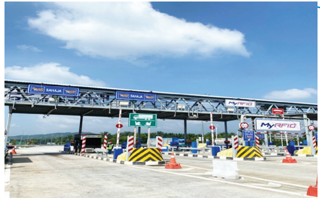
Fully electronic toll collection lane
