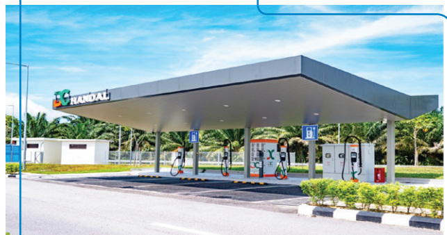
EV Charging Station at Trong Layby
