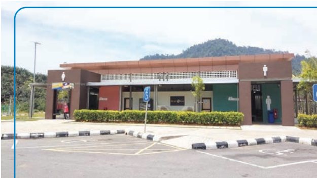
One of the RSA located at Sg Nyior (Southbound)
