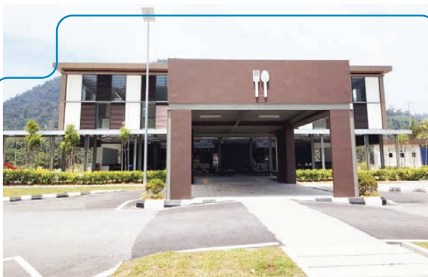
Sungai Nyior RSA (Southbound)
