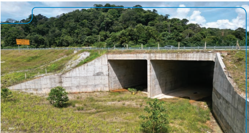
Animal box culvert at Section 11
