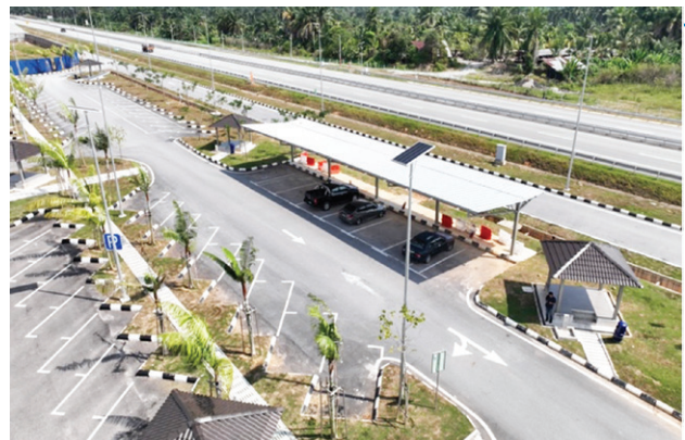
Solar lighting at RSA's parking area
