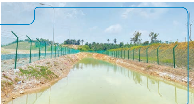
On site detention pond at RSA Section 6 Bukit Kapar (North bound)
