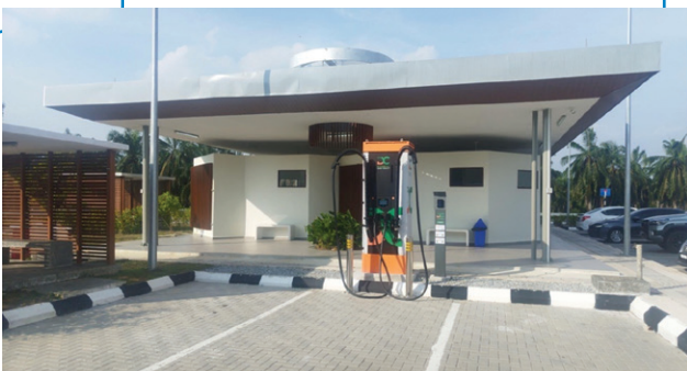
EV Charging Station at Assam Jawa Layby
