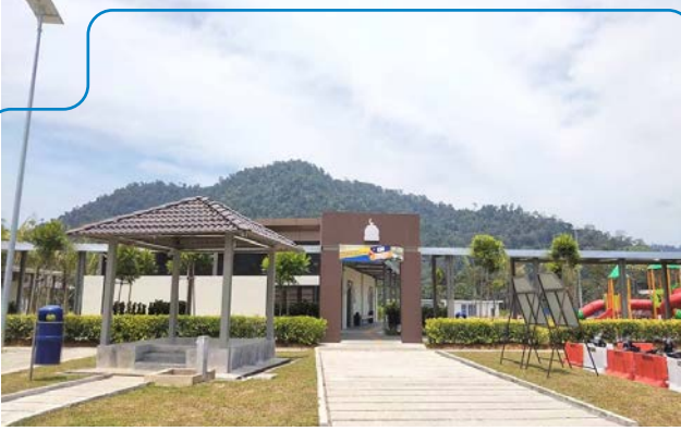
Sungai Nyior Rest and Service Area at Section 11 (Southbound-Northbound)
