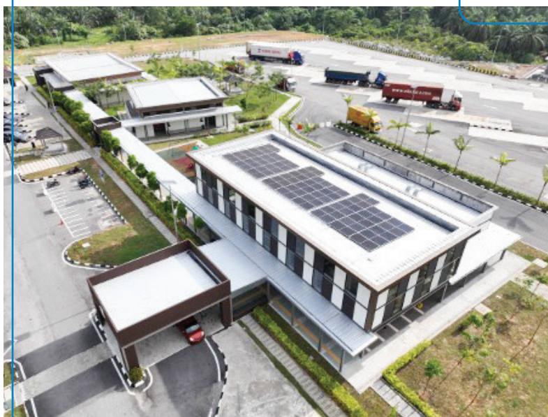
Aerial view of rooftop solar panel at RSA Sungai Nyior (Northbound)
