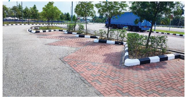
Permeable pavement at layby Bandar Bukit Raja Toll Plaza to control storm water runoff
