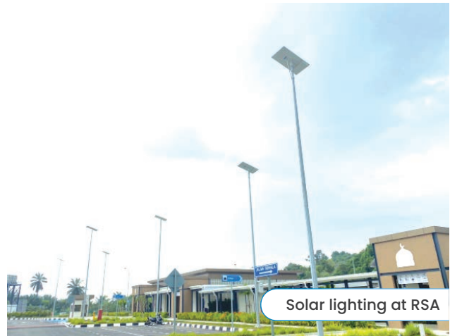
Sungai Nyior RSA (southbound)
