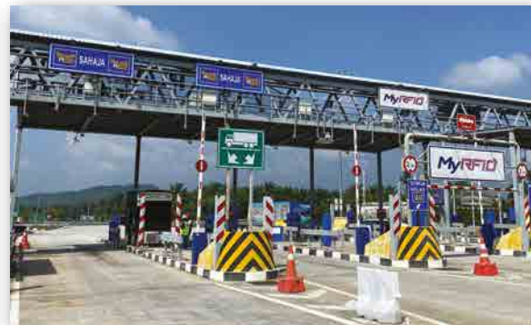
Fully Electronic Toll Collection via Touch n Go, SmartTag and RFID lanes
