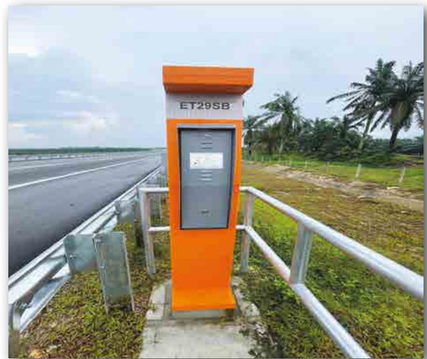
Emergency telephones are installed on both sides of the highway at every 2 km
