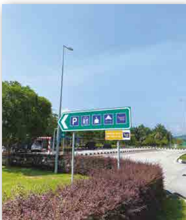
Lay-By with basic facilities (surau & toilet)
